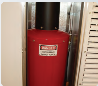
On-board water heater heats water to 71 °C for more aggressive cleaning
